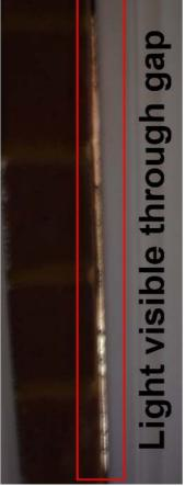
This is required unless there is existing sound mastic fully filling the gap to the frame surface with no light visible through the gap. Gaps with existing sealant not to the surface, defective or missing sealant must be fully filled.
