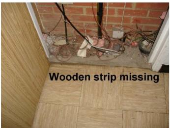
Fit a hardwood strip to the floor for the full width of the door frame extending from the front of the fire door to inside the inner edge of the door frame within the cupboard at a clearance of 2mm-3mm underneath the riser fire door (see image where properly fitted). Knot, prime and paint the new wood in colour black to match skirting.
